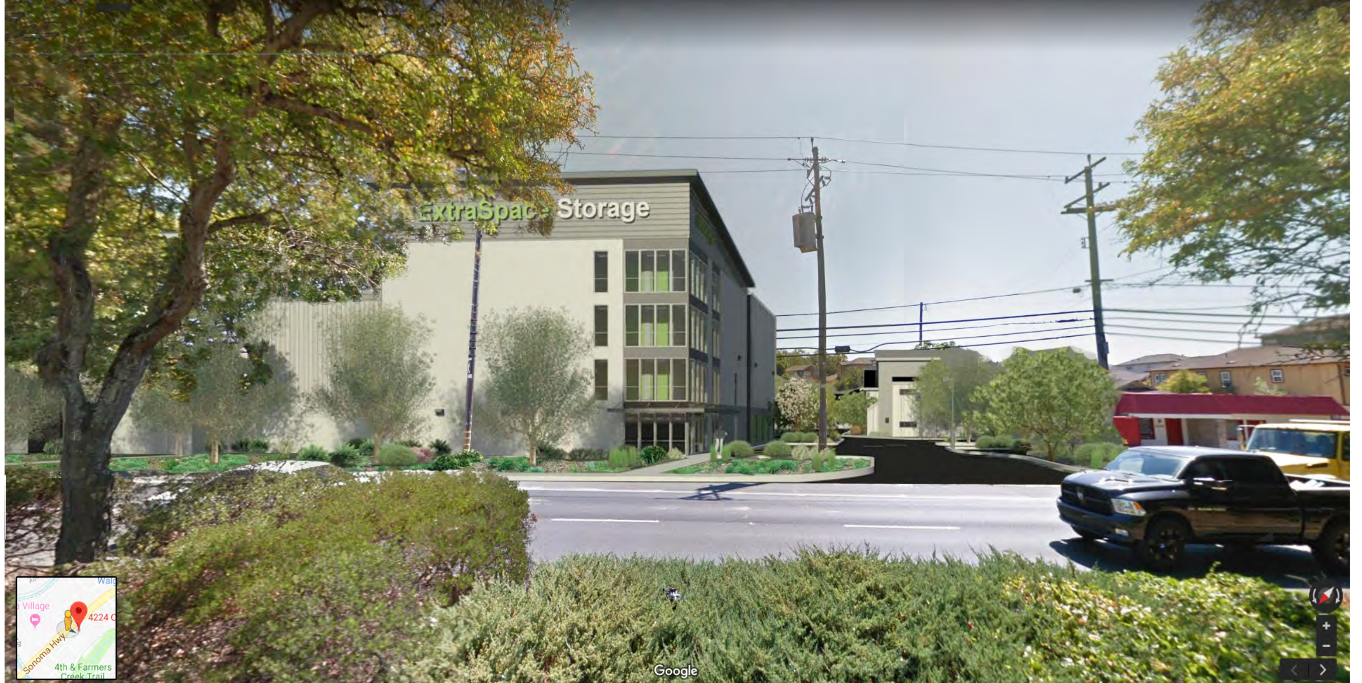
Recess Storage Project Santa Rosa, California
